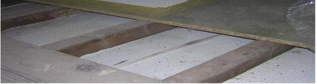
These slabs are relatively simple to install but must be cut oversize by 5mm between the joists to allow for a good friction fit. All joins and abutments must sealed with a compatible fire and acoustic acrylic sealant.
